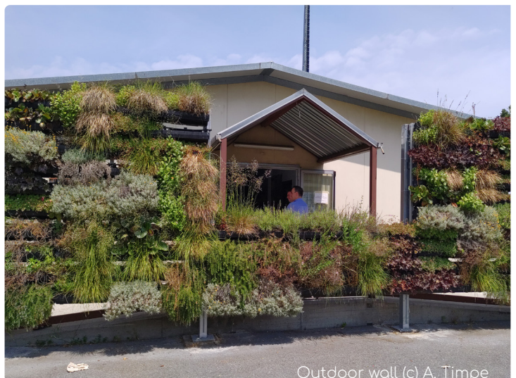
Outdoor wall (c) A. Timpe
